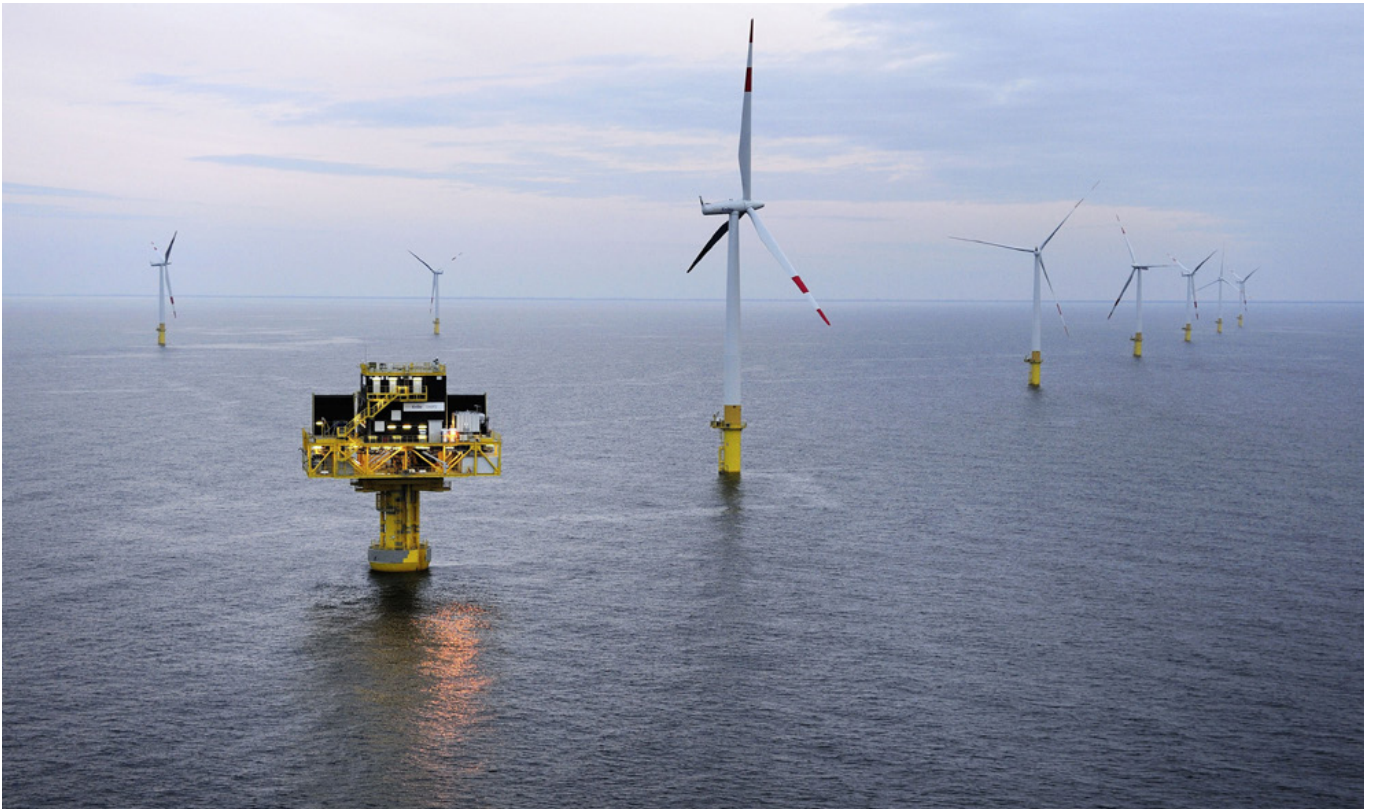
With ever more offshore wind capacity coming online in the North of Germany, grid stability is put to the test on windy days. Photo: 50Hertz (of Baltic 1).
