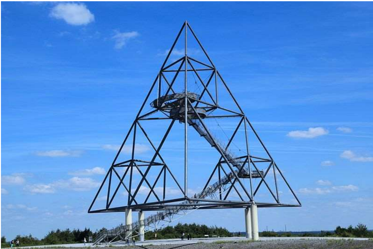
The Tetrahedron in Bottrop (German: Bottrop Tetraeder or officially Haldenereignis Emscherblick) is a walkable steel structure in the form of a tetrahedron with a side length of 60 metres, resting on four 9 metres tall concrete pillars. It is located in Bottrop, Germany, on top of the former coal mine dump Halde Beckstraße
